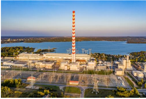
The Elektrėnai Complex:
